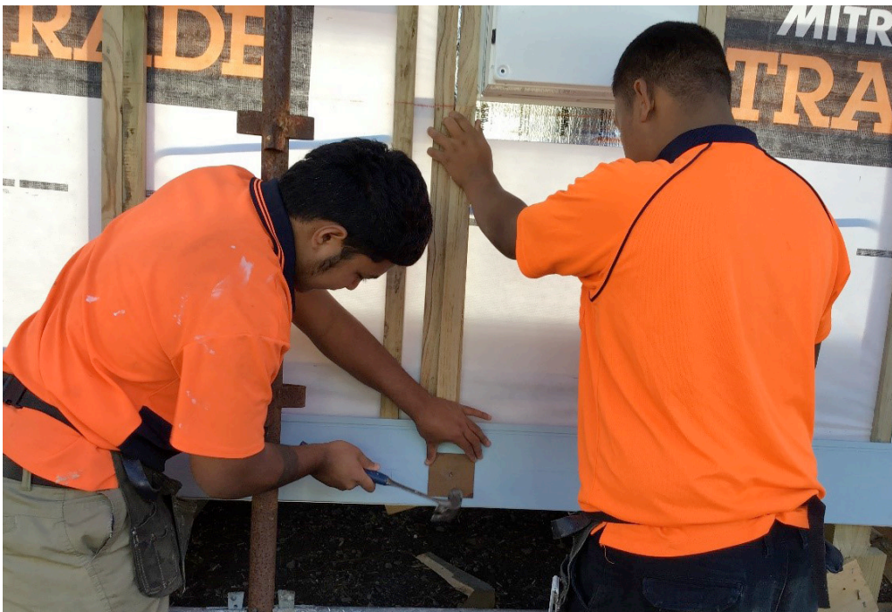
Students at Bay of Islands College constructing a house.
