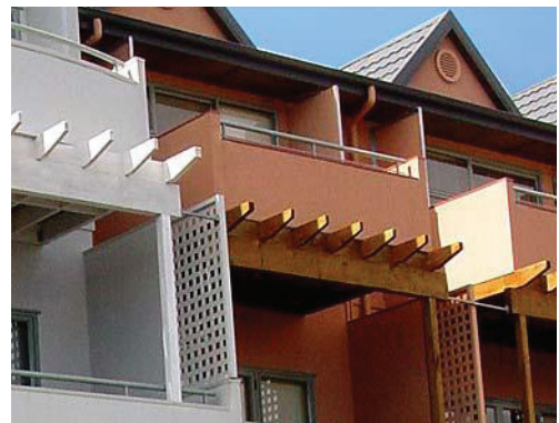
Fibre cement sheets as an exterior cladding
