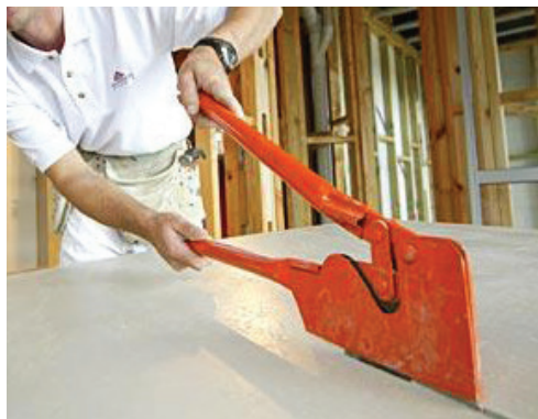
Cutting fibre cement sheets
