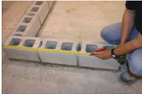
Measure 900mm along one side and mark the brick or block.
