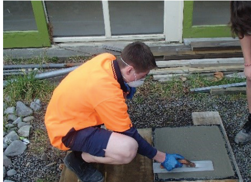
Double checking the paver's thickness.
