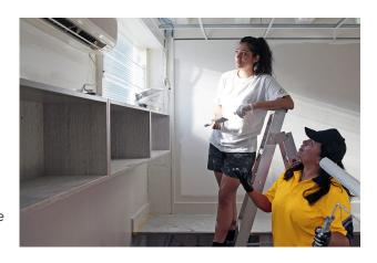
Painters and decorators need good maths skills. They need to calculate the amount of paint needed for an area to purchase enough in one batch, which is important for colour consistency. They need to know ratios for mixing wallpaper paste and for diluting paint according to manufacturer's recommendations.
