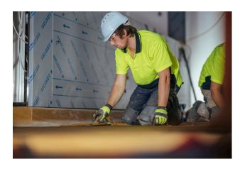
Resin flooring applicators apply specialist resin flooring systems. Resin floors are made by mixing together ingredients that have a chemical reaction. The chemical reaction produces a durable and safe protective surface on concrete.
