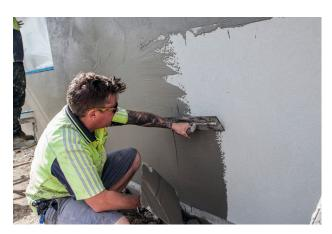
Exterior plasterers are sometimes simply known as plasterers. They mix and apply plaster to form the exterior cladding of a building, or to form smooth or textured surfaces for pools and walls.
