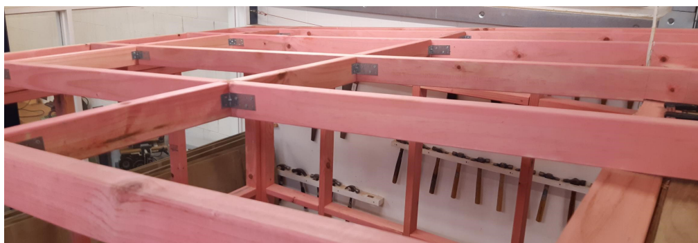
Completed roof framing
