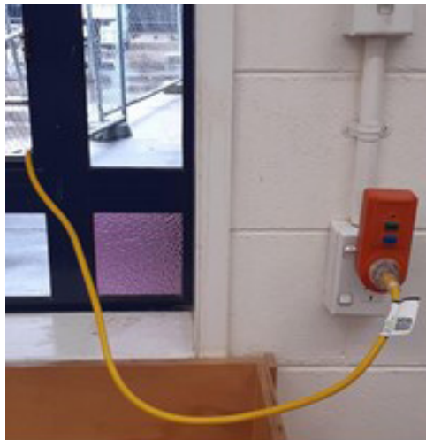
Use a residual current device (RCD) if working outside no matter what the weather conditions are
