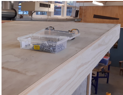
17mm CD plywood roofing being fitted
