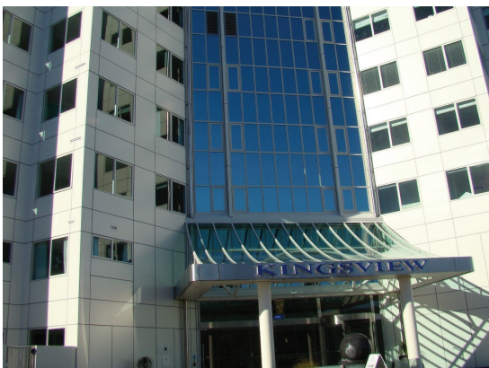
Several types of glass may be needed for one building
