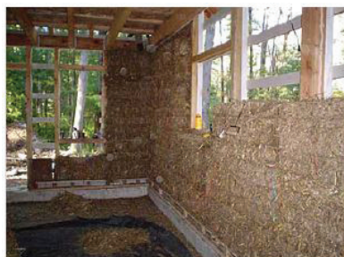
Straw bale house being constructed.
