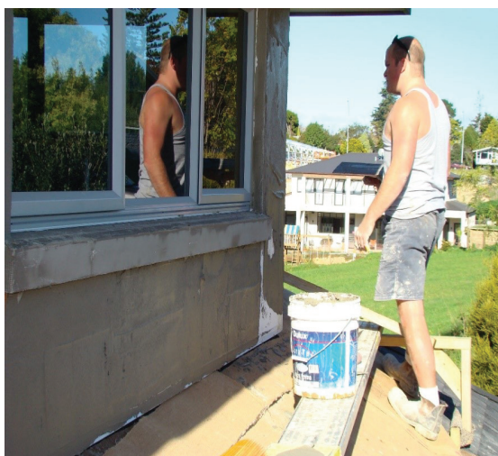
The plasterer finishes off the external cladding once the joinery is installed.
