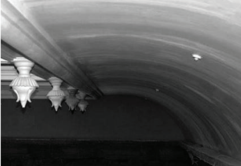
Concave sheets installed and ready for finishing.
