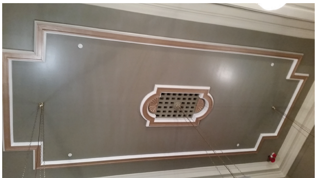
Cornices and decorative mouldings, made by fibrous plaster manufacturer, and installed then finished in this ceiling by an interior linings finisher.
