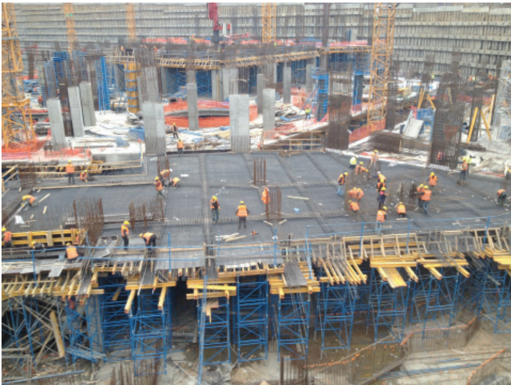
Falsework supporting the structure before concrete is poured to form the floor.
