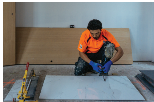
Getting tiles ready to set out
