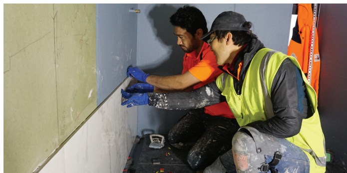
Fixing wall tiles
