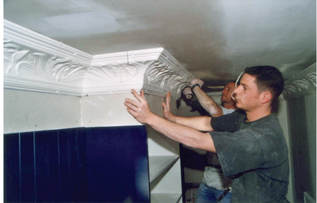
Fibrous plaster cornice and decorative mouldings are fixed using a combination of mechanical fixings and a special plaster mix. The fixing and finishing of cornices requires internal and external mitred corners. Special care must be taken to match pattern designs with repetitive features.
