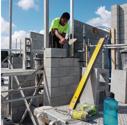
Masonry block walls being constructed.
