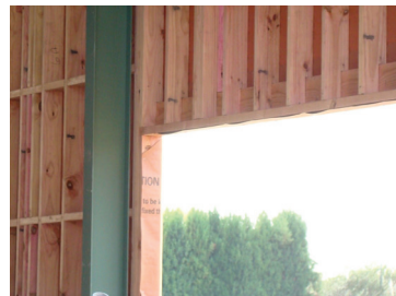
Space created for the window to be installed.
