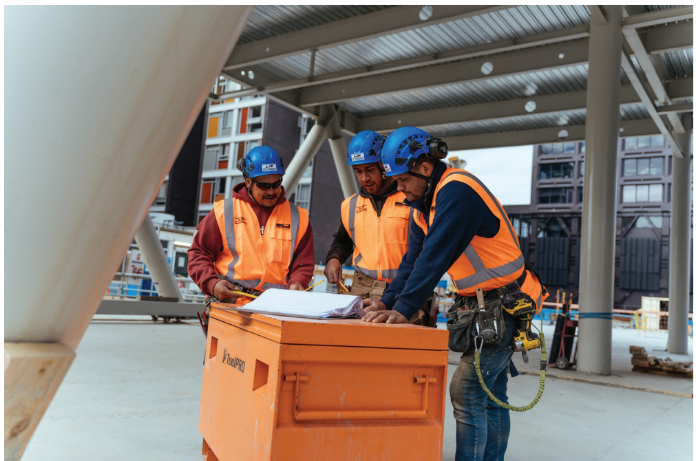
Checking plans and specifications on site.
