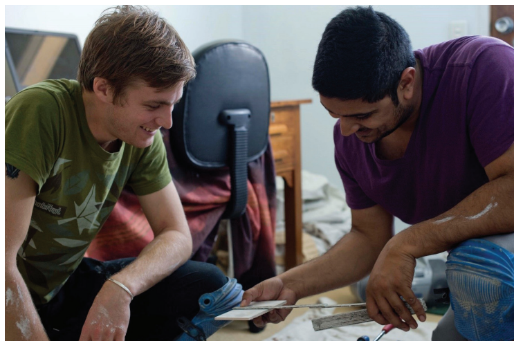
Double-checking the tile was cut to the correct size.
