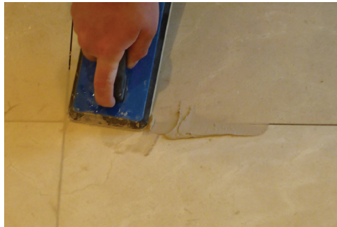
Applying grout
