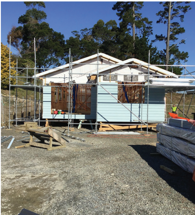
Bay of Islands College's BCATS students' relocatable house in the process of being constructed.
